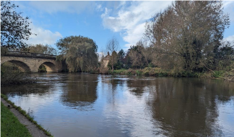
Figure A.38: Swinford toll bridge
