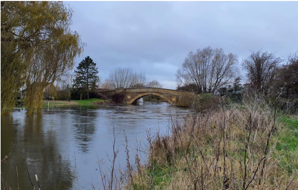
Figure A.32: Tadpole Bridge over the River Thames
